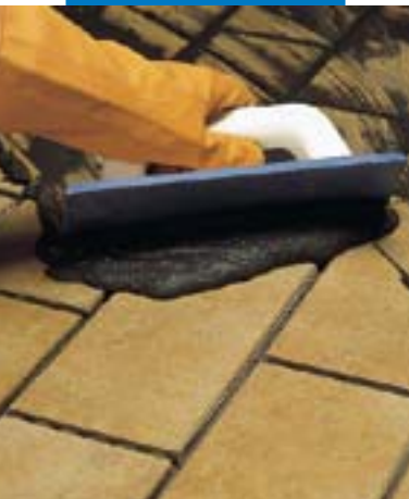
Grouting an external klinker tile floor with Keracolor GG mixed with Fugolastic
