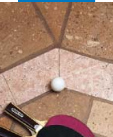
Terracotta floor polished in situ, grouted with Keracolor GG mixed with Fugolastic
